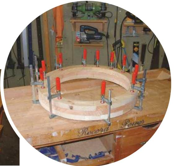
▲ Pic.7 Apply glue to all surfaces and cramp the third layer to the frame. Clean up when dry
